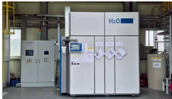
Vacuum Evaporation and Concentration System for Waste Oil at Seosan Plant
